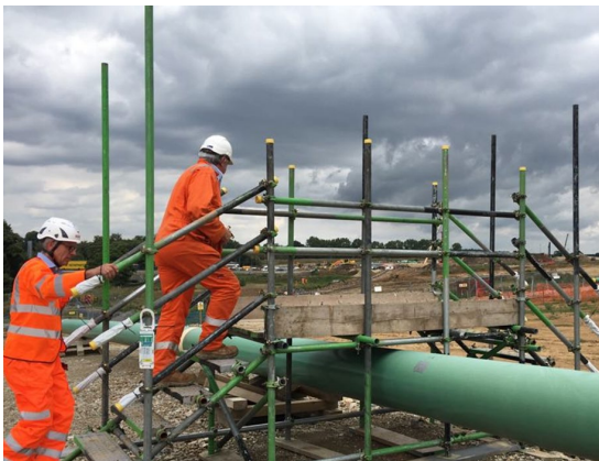
Photo 3.1: Indicative temporary steps over pipe string (pipe larger than SLP pipeline)
